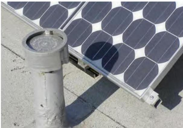
Figure 11: Vent pipe shadow
