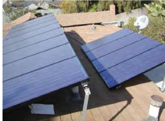
Figure 10: Row to Row Shading
